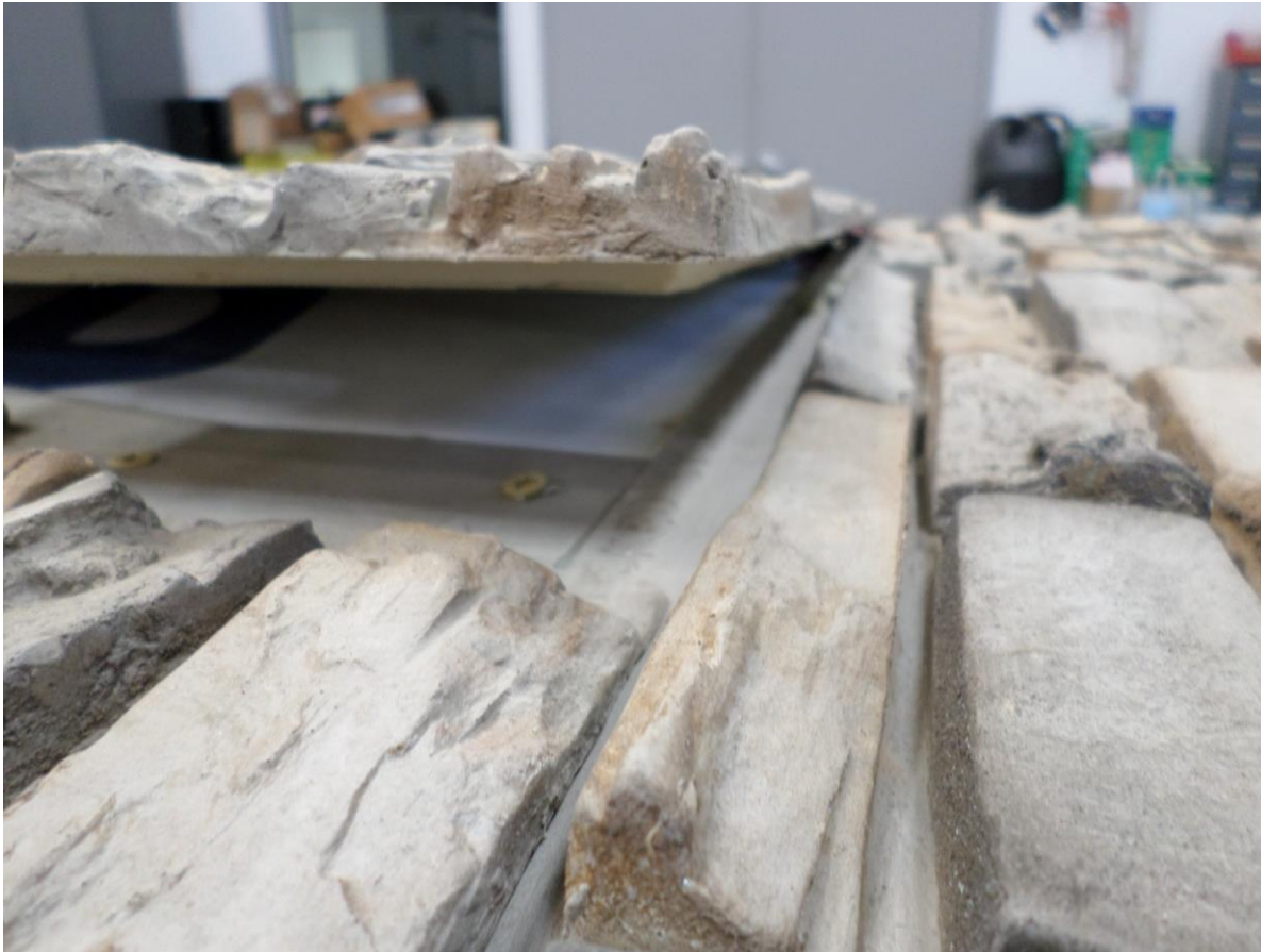
Photograph No.3 Typical results of the negative load test Tongue and groove failure
